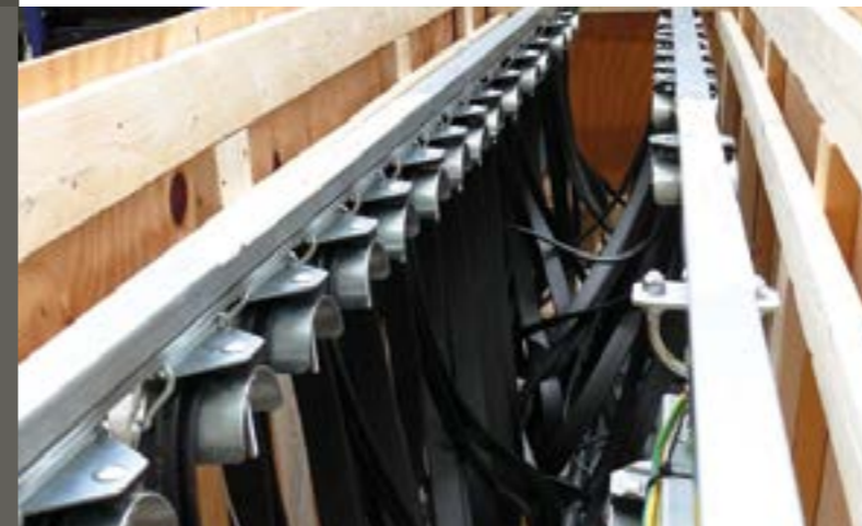
Prewired hoist trolley power supply
