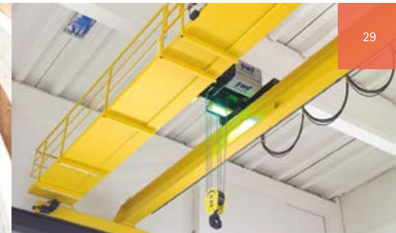
Double girder overhead bridge crane with crane lights
